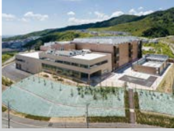
Data Center Operation (Japan) MC Digital Realty, Inc. A Data Center Operation Joint Venture with Digital Realty Trust
