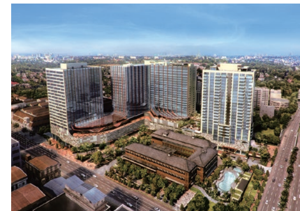
Yoma Central Project in Myanmar
